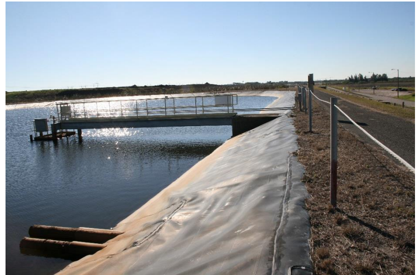
Economizer Ash Suction Pond (west side, looking south at instrumentation platform )
