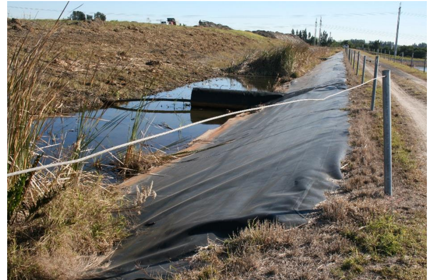
South Economizer Ash Pond (south side, looking east)
