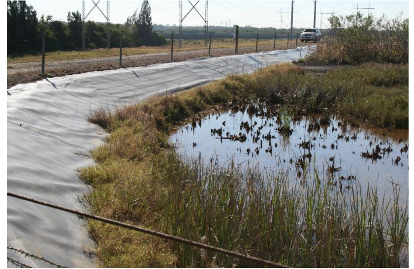
North Economizer Ash Pond (east side, looking south)
