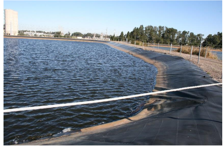
Economizer Ash Suction Pond (east side, looking northeast)
