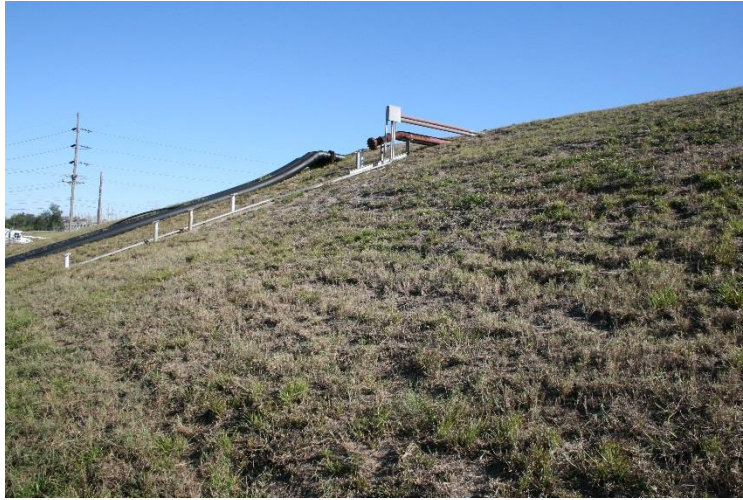
Economizer Ash Suction Pond (west side, looking east at embankment penetrations)
