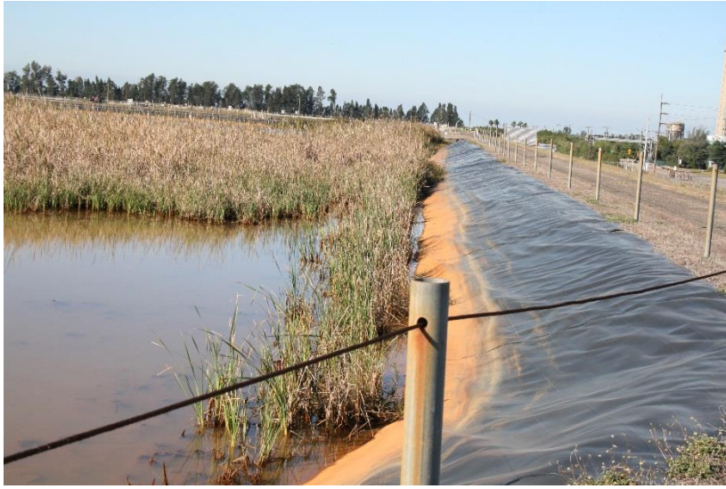
North Economizer Ash Pond (north side, looking west)
