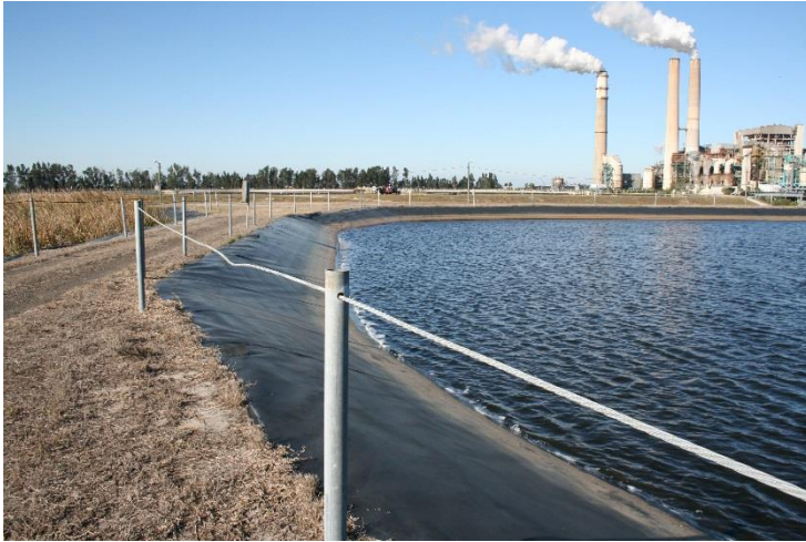
Economizer Ash Suction Pond (south side, looking west)
