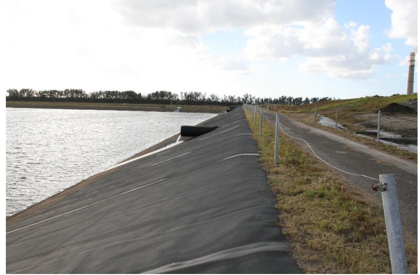
South Economizer Ash Pond (south side, looking west)
