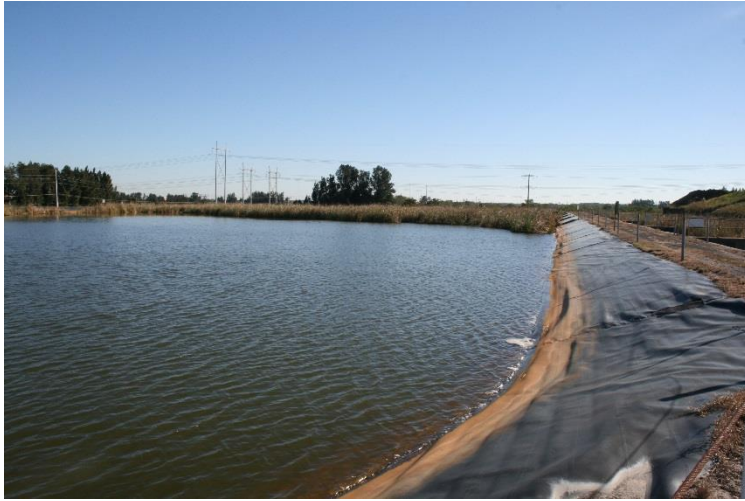
North Economizer Ash Pond (south side, looking east)
