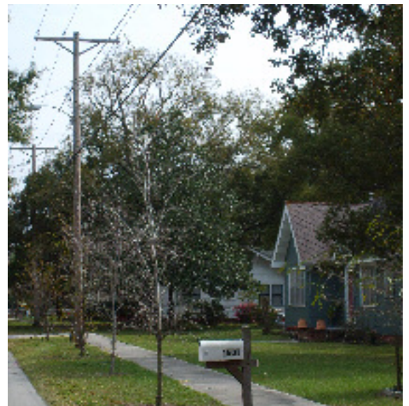
Overhead electric service to a residential building.
