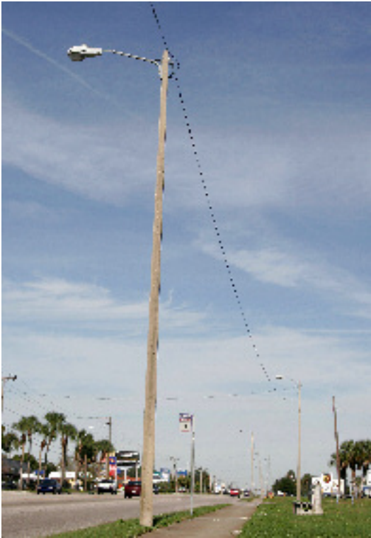
Overhead system street lighting.
