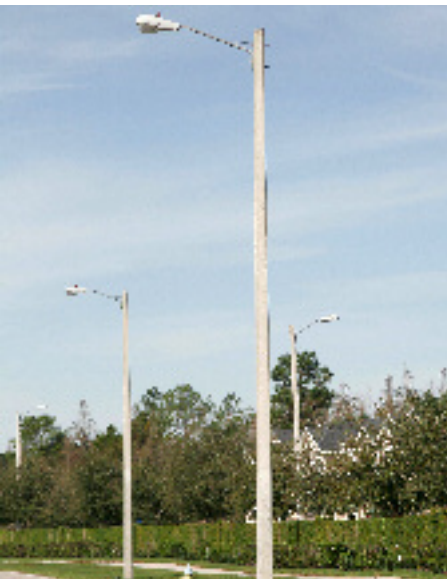
Underground system street lighting.
